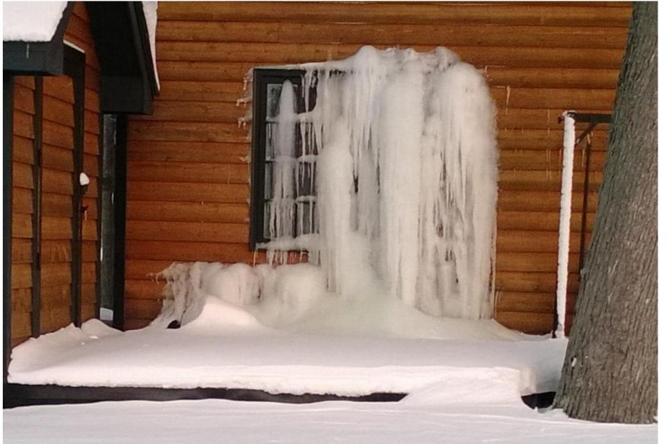
A blocked intake on dual pipe 90% furnace caused this No Heat situation
